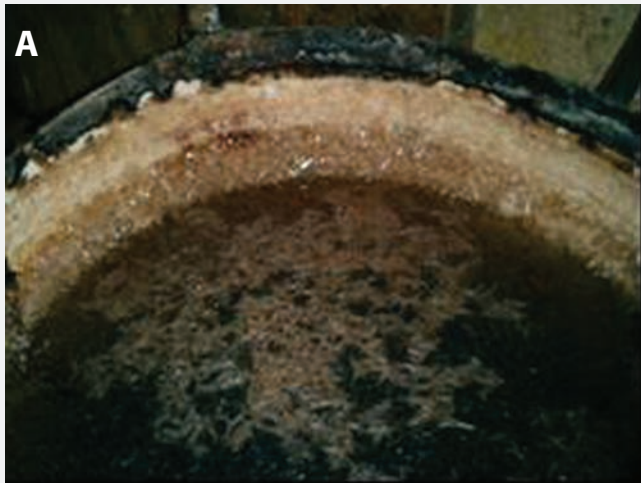
Figure 1: Water-soluble product precipitation in stock-solution containers that resulted in clogged medicator input lines. A: Container completely lined with crystals and black sludge. B: Container completely lined with white crystals, with precipitated product floating. C: White precipitate throughout the solution. D: Precipitated product floating.
